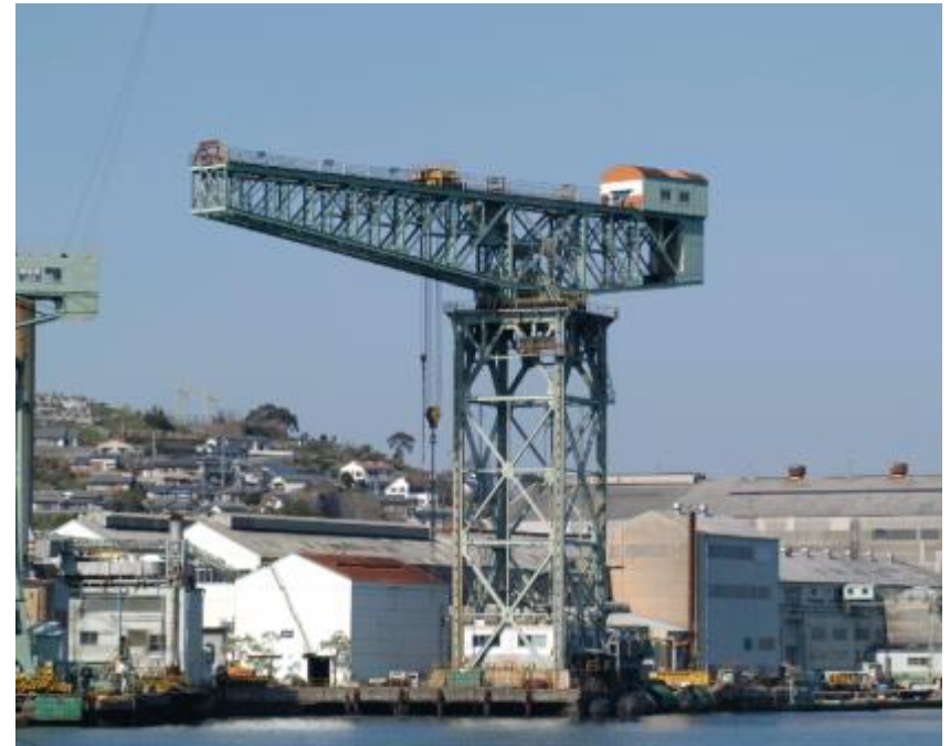
World Heritage: Giant cantilever crane
