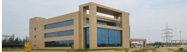
Kattupalli – Admin Building
