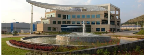
LTSSH – Admin Building
